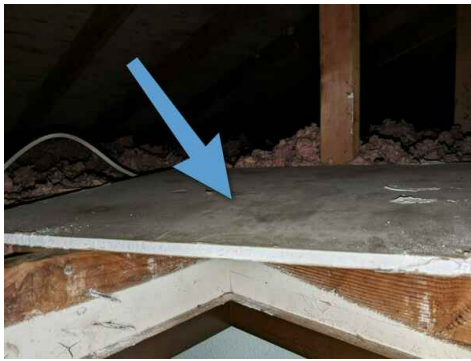
missing insulation
